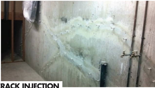
CRACK INJECTION
