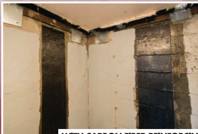
WITH CARBON FIBER REINFORCING
