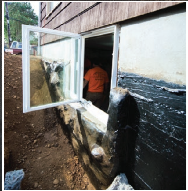
SALEM CONFERENCE CENTER EXTERIOR BRICK WATERPROOFING
